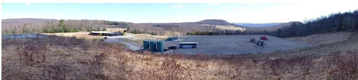
Figure 3 Overview of active gas production wells on a well pad
